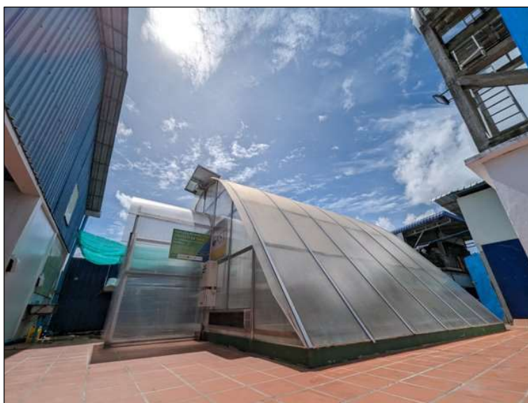
Figure 2: Large-scale solar dryer dome suitable for medium to large sized processors
